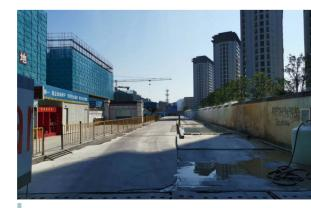
Passage of washing equipment for construction vehicle
