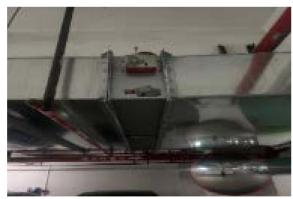
On-Site Pictures of the Replacement of Fire Smoke Exhaust Dampers
