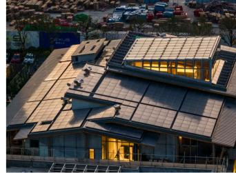
Gray Monocrystalline Silicon Photovoltaic Panels
