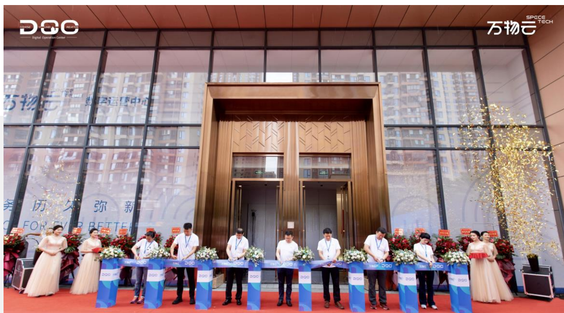
Official Opening of Wuhan Digital Operation Center Building
