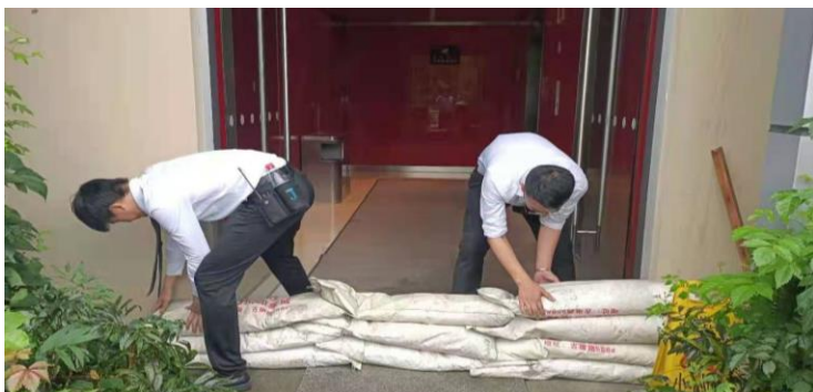
Utility of sand bags to reinforce the defense line to prevent the flooding
