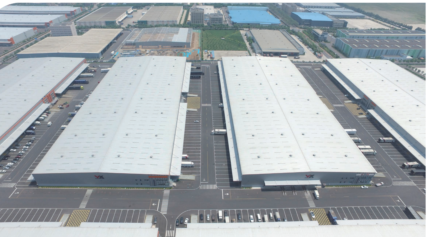
Logistic and Warehousing – Dayaowan Project in Dalian
