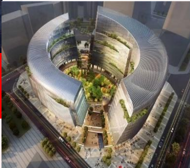
Chengdu High-tech Vanke Center (internal referral) Total contract area: 151,800 sq m
