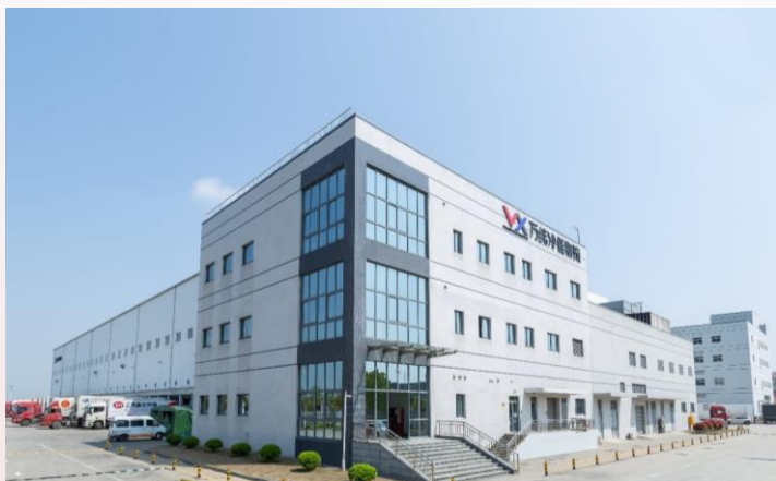
VX Shanghai Haigang Cold Chain Logistics Park
