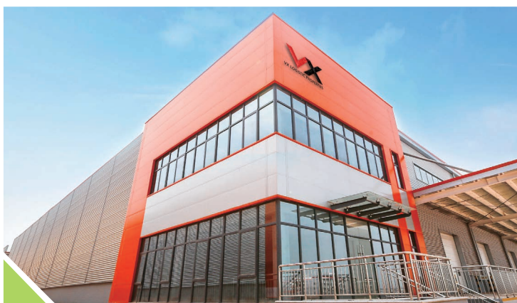
Wuhan Yangluo Warehouse
