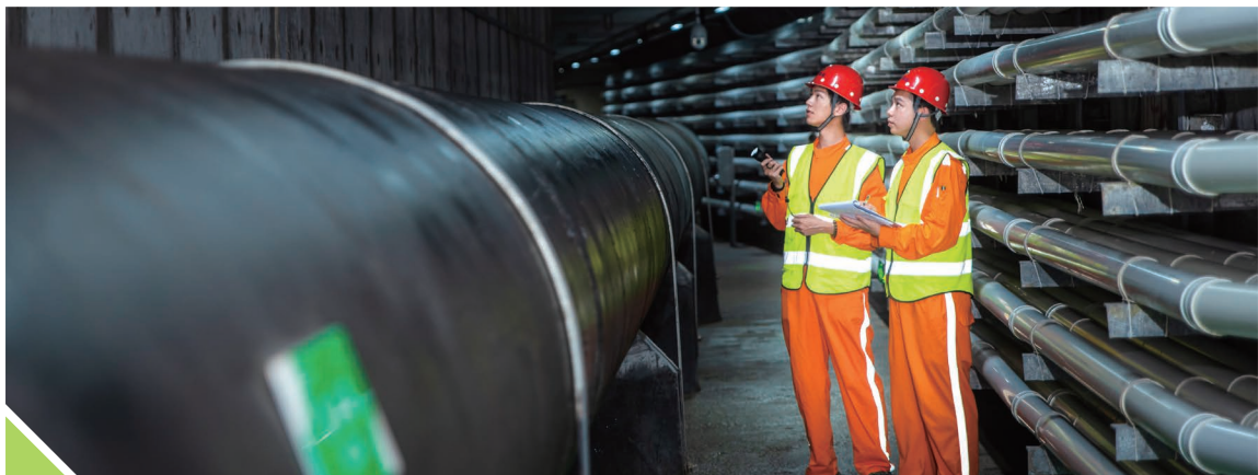
The underground comprehensive pipeline corridor located in Hengqin is 33.4 kilometers long. This photo shows staff carry out daily inspection inside it.
